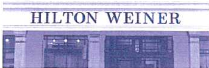
Figure 24: Nineteenth-century style lettering successfully applied to the fascia of a colonnaded verandah.
